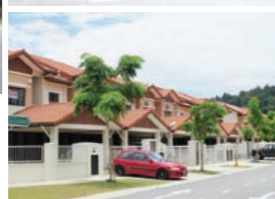
142 units of 2-Storey Superlink Homes @ Precinct 2A handed over in 2009
