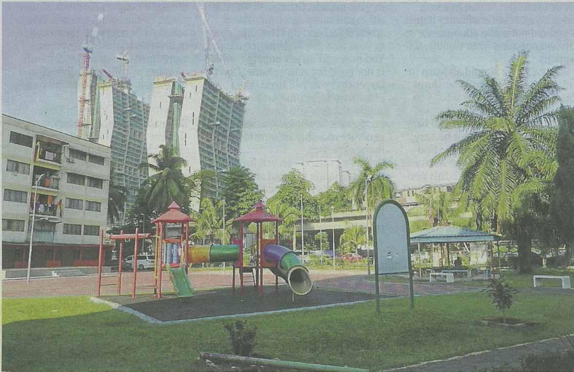
Provision of open and green spaces. The approval governs on how these open spaces allotted for the designated community activities such as playground for children, communal park, etc are to be used.
